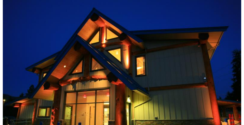
Quilakwa Center — Featuring huge cedar columns and crooked Douglas Fir collar beam. Photographer, Peter Sperlich. Photo courtesy of Wood Design & Building Awards.
