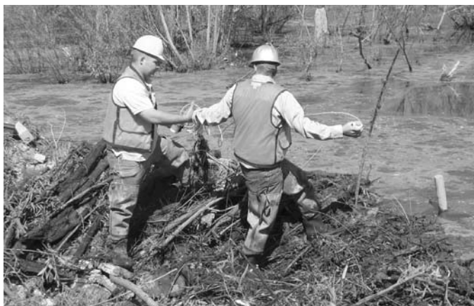
BMAP staff prepare to demolish a beaver dam.
