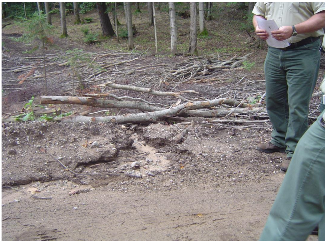
Slash ineffective in controlling run-off from road
